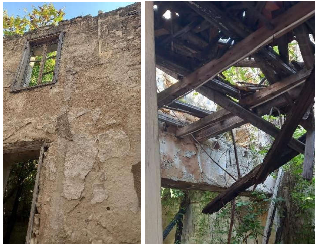
Figure 4. Damage to the walls and interior of building B
