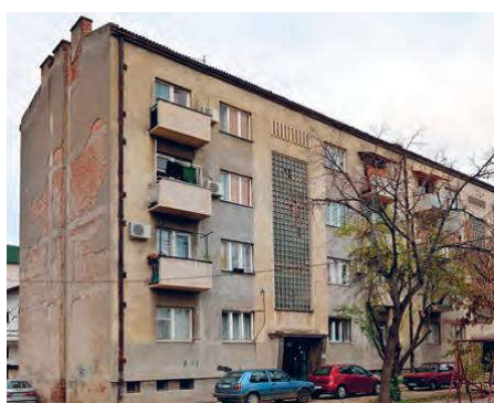
Figure 2. A residential building with load bearing facade brick walls without thermal insulation [3]
