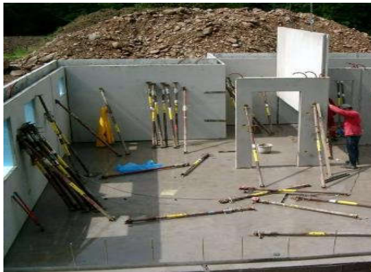
Figure 2. Precast concrete Twin Wall [28].
