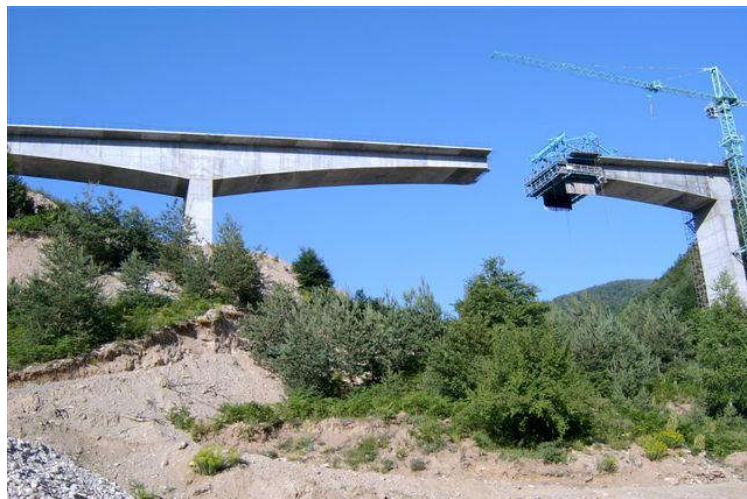
Figure 2. Cantilever construction of "Makaza" viaduct [8]
