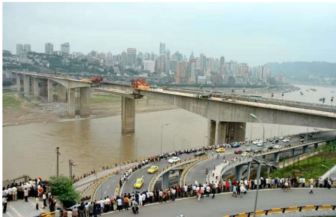
Figure 1. Road bridge "Shibanpo", China [7]
