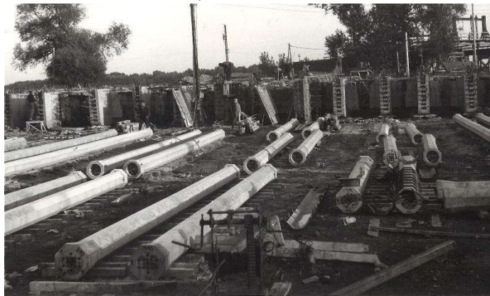
Figure 2. Pre-assembled hangers at the place of manufacture [4]
