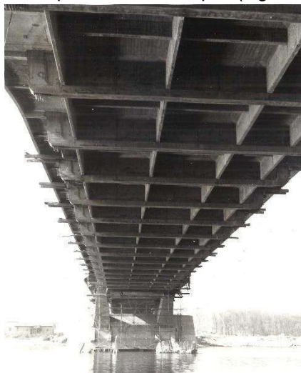
Figure 3. Track plate and secondary supports [5]
