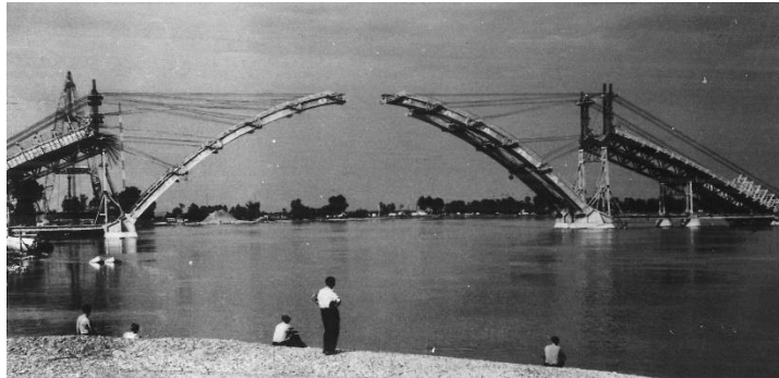
Figure 6. Installation of arched scaffolding of a large arch [5]
