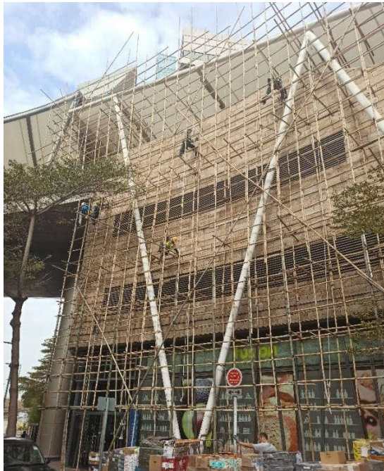
Figure 5. Bamboo scaffolding (photo taken by author)
