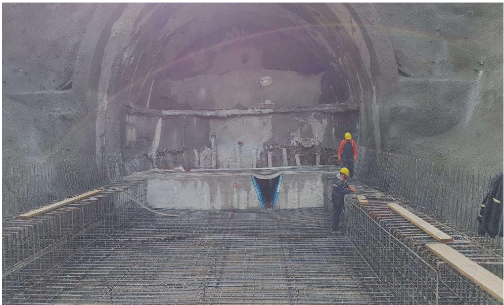
Figure 3. Formation of cut and cover section in the right exit portal of the Kosman tunnel in a length of 10m
