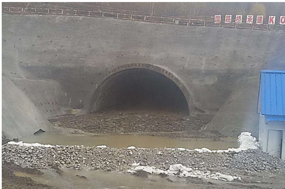
Figure 1. The soil that filled the right exit tube of the Kosman tunnel after the collapse of the excavation face
