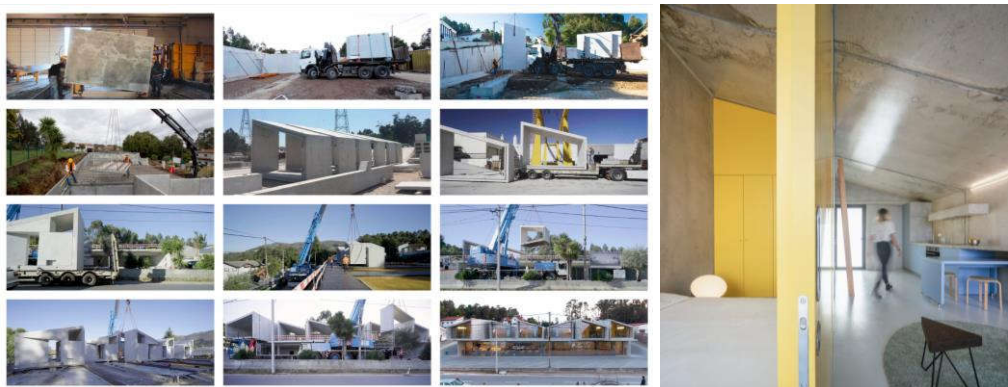
Figure 8. Phases of construction process – fig. 8 – left; internal problems with the connections between elements – fig. 8 - right, source [11]
