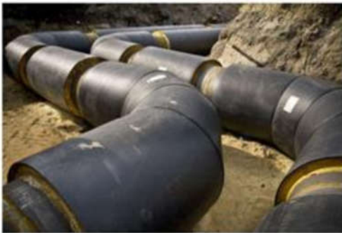
Figure 5. Usual size of the piping within the geothermal system based on hot water, Iceland, www.verkis.is , presentation by T. Johannesson at Cornell, 2016
