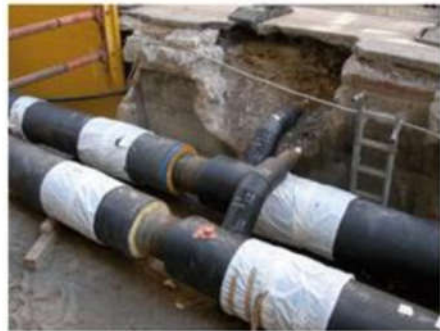
Figure 5. Usual size of the piping within the geothermal system based on hot water, Iceland, www.verkis.is , presentation by T. Johannesson at Cornell, 2016
