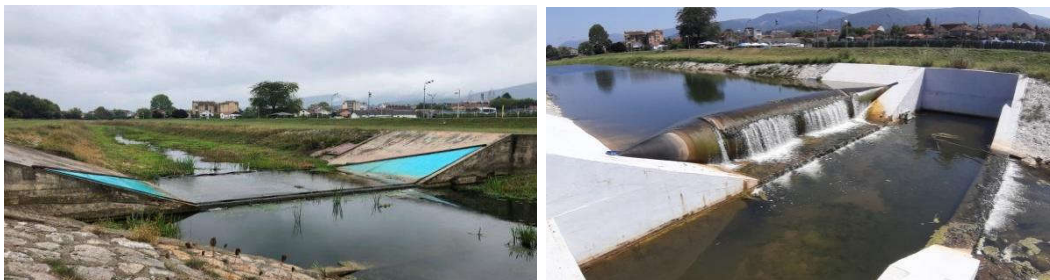
Figure 4. Before and after inflatable dam installation in the City of Svrljig
