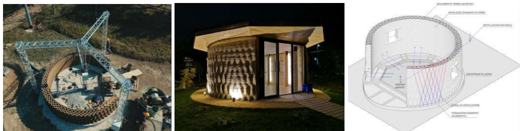
Figure 3. First 3D house printed with soil material, „Gaia“, 2018 [5]
