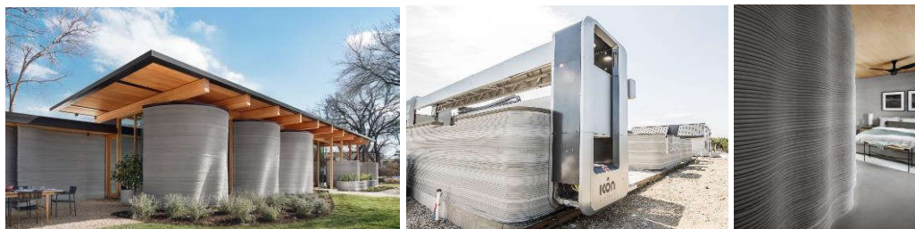
Figure 4. Companies ICON and LAKE FLATO built a 3D printed house Zero in Austin, Texas, 2022 [7]
