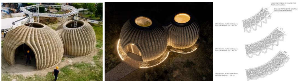
Figure 2. 3D-TECLA, first printed biomorphic mud cottage built in Ravenna, Italy [3]
