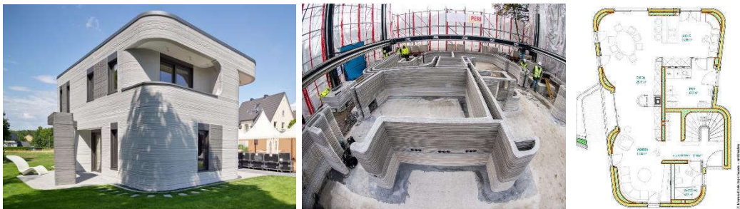
Figure 6. Beckum, Germany, features the first 3D printed two-storey building, 2021 [11]
